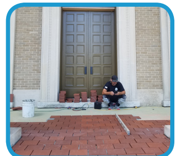
Terra cotta pavers were removed and replaced on both landings, including a new, upgraded setting bed and new mortar joints throughout.
