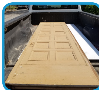
Each door leaf was taken off-site for repair and refinishing.
