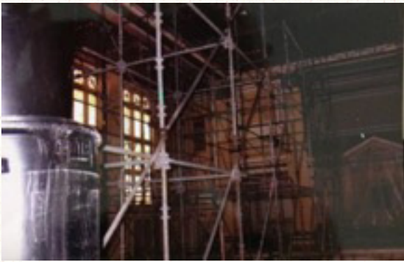
OST sanctuary under repair 2004-2005
